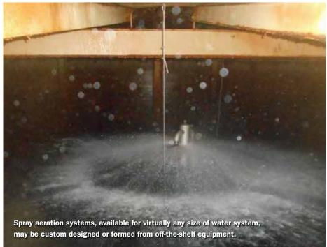
thereby ensuring no untreated water can flow into and out of the tank without being treated.
