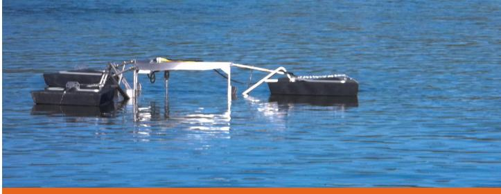
Floating wastewater mixers are a proven odor control strategy for many types of wastewater ponds and basins.
