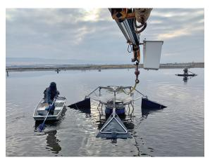
One of four SolarBee mixers being installed using a crane at the Grandview lagoon.
