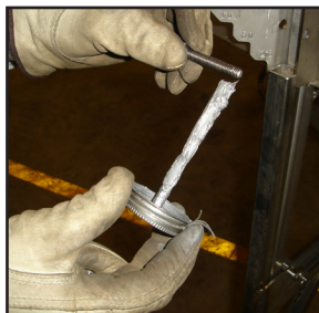
Applying Anti-Seize To The Bolts
