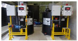
lxom Bullet<sup>™</sup> self-bunded chemical dosing system (no requirement for expensive concrete bund)
