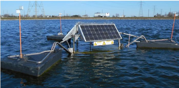
exit the pond much easier (as usually evidenced by up to 300 methane bubbles per square meter) across the entire lagoon. The increased methane release speeds up anaerobic digestion of bio-solids at the bottom. Better & more effective sludge reduction eliminates any need to ever dredge the ponds.
