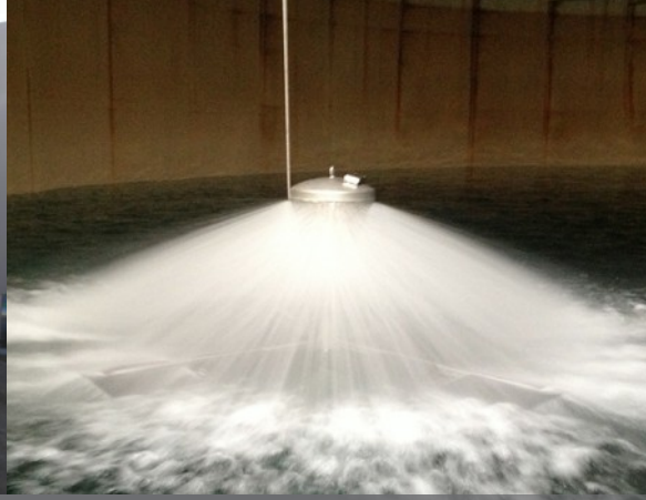
One of the three tanks, SN15 GridBee® Floating Spray Nozzle THM Removal System, and blower assembly
