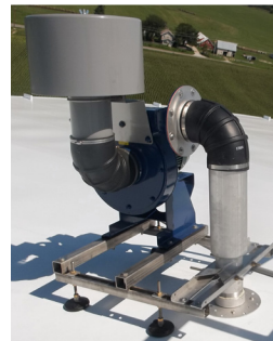
Headspace Ventilation , designed to meet project needs
