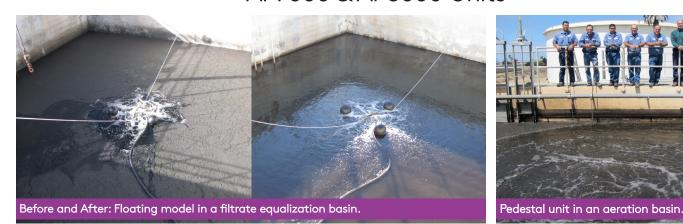
GridBee® AP Air-Powered Mixers from Ixom Watercare combine patented long-distance circulation technology with a clog-free design. These powerful mixers are compact, portable, can be used at any depth, and are easy to install.
